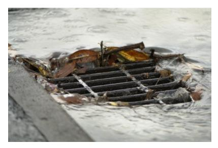
and natural conveyance in the form of infrastructure such as creeks, culverts, detention basins, drywells, pipes, localized treatment systems, and storm drain inlets. This infrastructure collects stormwater, and in some instances partially treats it, before the stormwater is discharged to either groundwater or surface water.
