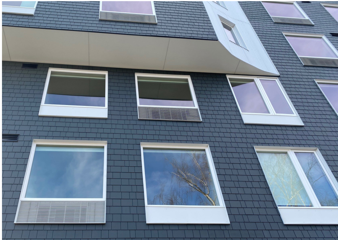
PRECEDENTS: FIBER CEMENT SHINGLE SIDING WITH PROTRUDING METAL WINDOW TRIM
